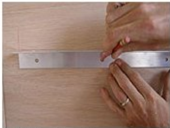
(1.) Select location, mark holes
