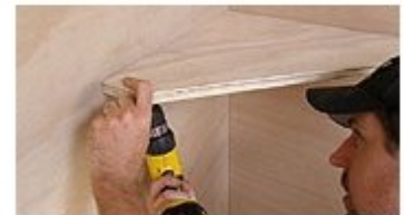
(6.) Fasten screws through brackets into shelf
