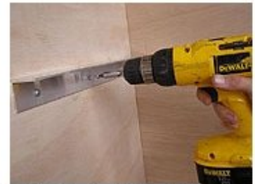
(3.) Fasten both brackets (level) against corner walls level with adjacent bracket
