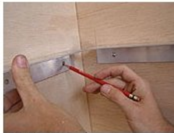
(2.) Mark both angle brackets level with adjacent bracket
